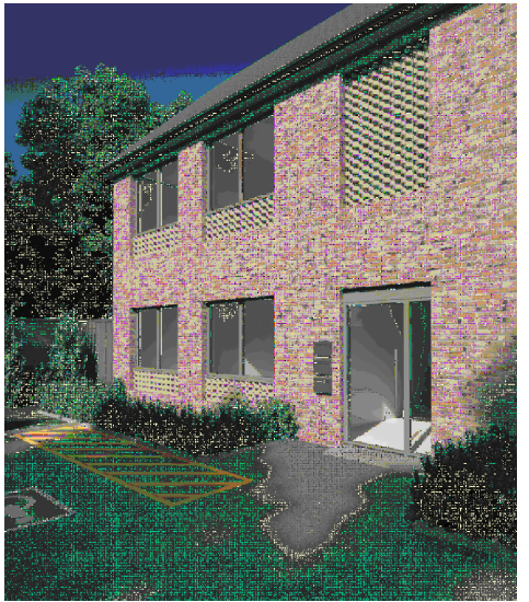
EXAMPLE: YELLOW LONDON STOCK BRICK AND TOOTHED BRICK FORMATION
